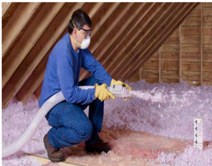
Figure 1. Insulation being installed in the attic of a home. Source: Attic Air website, 2016
